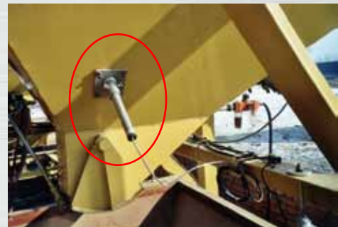
...same FSA probe (sight: from outside the silo)
