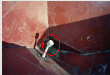
Arm - probe FSA in a Silo
